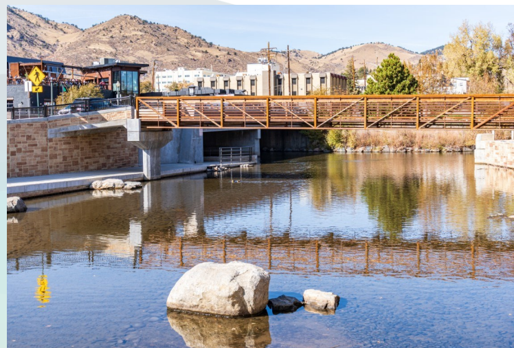
Now a recreational amenity, this greenway also protects over 1 million SF of industrial property from storm flows
