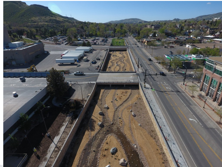
Kennys Run Greenway, post construction overview
