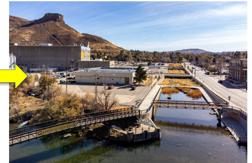
...To an open channel amenity providing a symbolic confluence of a historic City with a modernized brewery.
