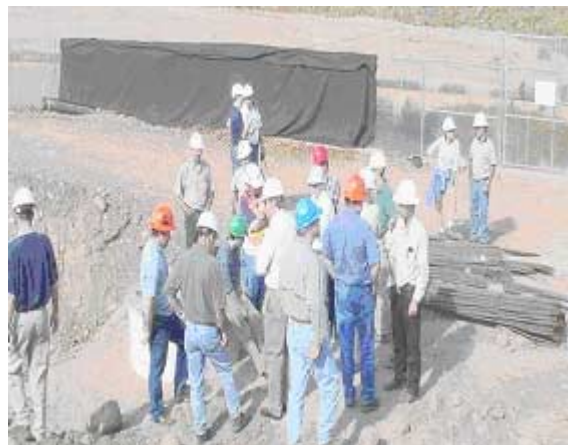
HORSETOOTH DAM – Members learn about installing a grout curtain centered in the existing embankment extending down more than 100 feet.
