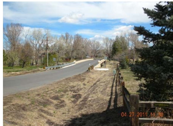
Caley Drive - After
