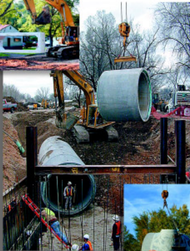
▲ Installation of 108-inch diameter RCP approaches the transition/drop structure.
