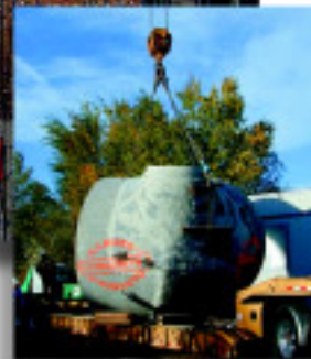
▲ 45 special fabrications were used on the project, including this 83-degree bend.
