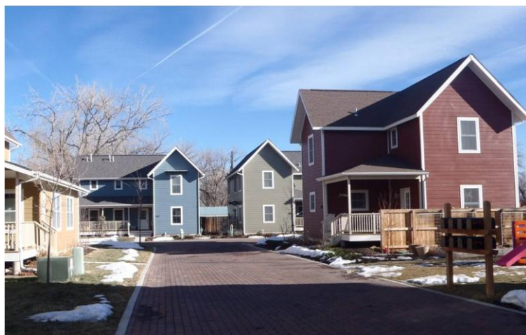
Photo 1. Toby Lane Development in Boulder protected from flood damage in September 2013 because the homes were elevated two feet above the 100-year flood elevation.
